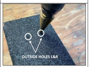
**STEP 4** REMOVE THE DRILLING TEMPLATE AND ENLARGE OUTER HOLES (L&R) TO <u>5MM</u>.
