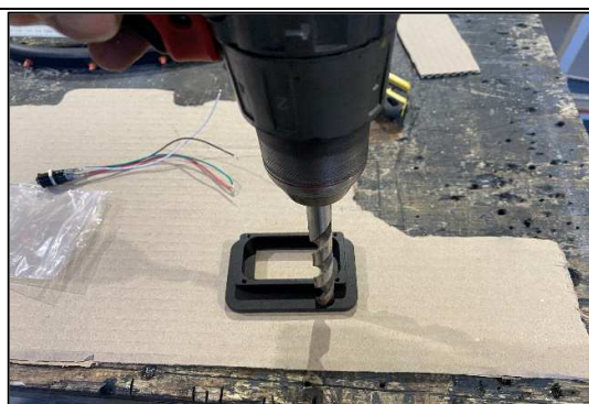
STEP 1.2.2 PLACE THE JBA FASCIA ON A SOFT SURFACE SUCH AS SOME CLEAN CARDBOARD. USING A 12MM DRILL, BEGIN DRILLING SLOWLY UNTIL A SMALL HOLE BEGINS ON THE FRONT SIDE.
