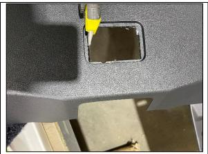
**STEP 1.7** TRIM THE MARKED OUT SECTIONS WITH A STANLEY KNIFE AS SHOWN. TAKE CARE NOT TO SCRATCH THE TOP SURFACE WHILE CUTTING.
