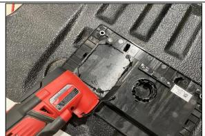
**STEP 3.1.3** FLIP PANEL OVER AND CUT OUT SECTION AS SHOWN.
